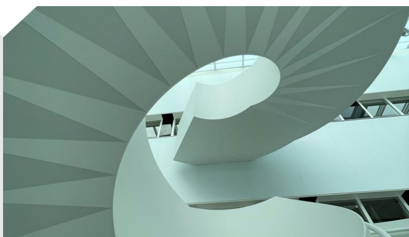
Image © Staalservice Hardenberg Detail of the spiral staircase
